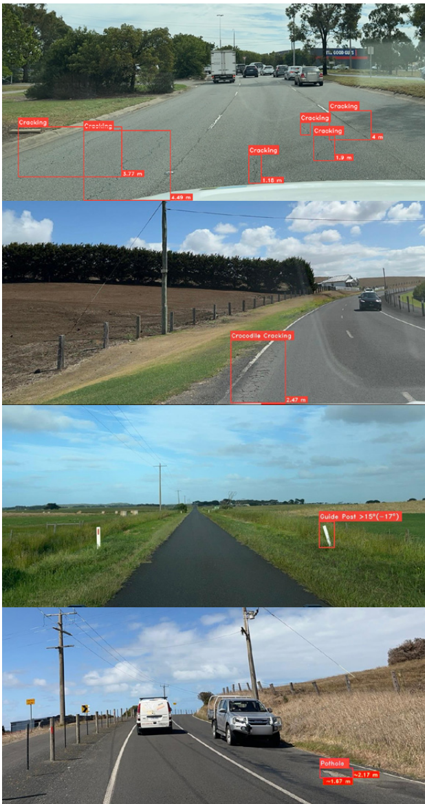
Example AI detected defects
